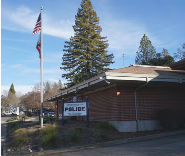
CITY OF PLACERVILLE Public Safety Building
