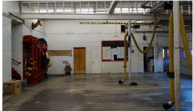
View of apparatus bay toward lobby
