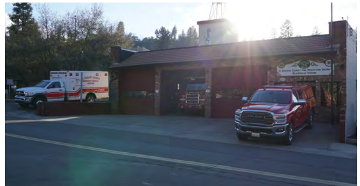
View of Station 25 from Sacramento Street
