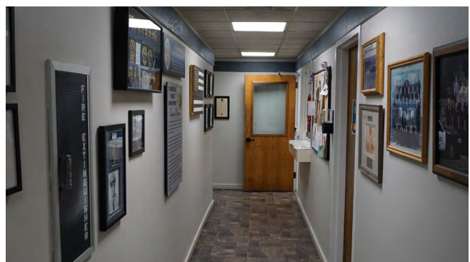
Typical narrow building corridors
